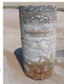
Core from N12 section showing asphalt and ETB base ►
