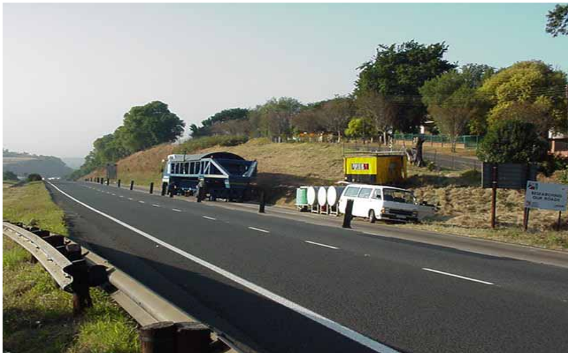
Picture 2.1: Site selected for HVS testing at km 16.3 N3 north bound
