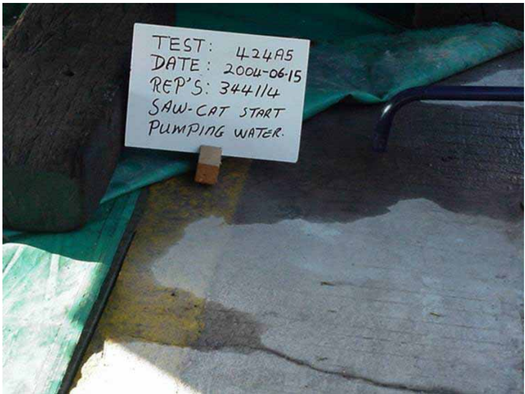
Picture 5.6: Clean water pumping out of longitudinal saw-cut edge after 344 114 repetitions
