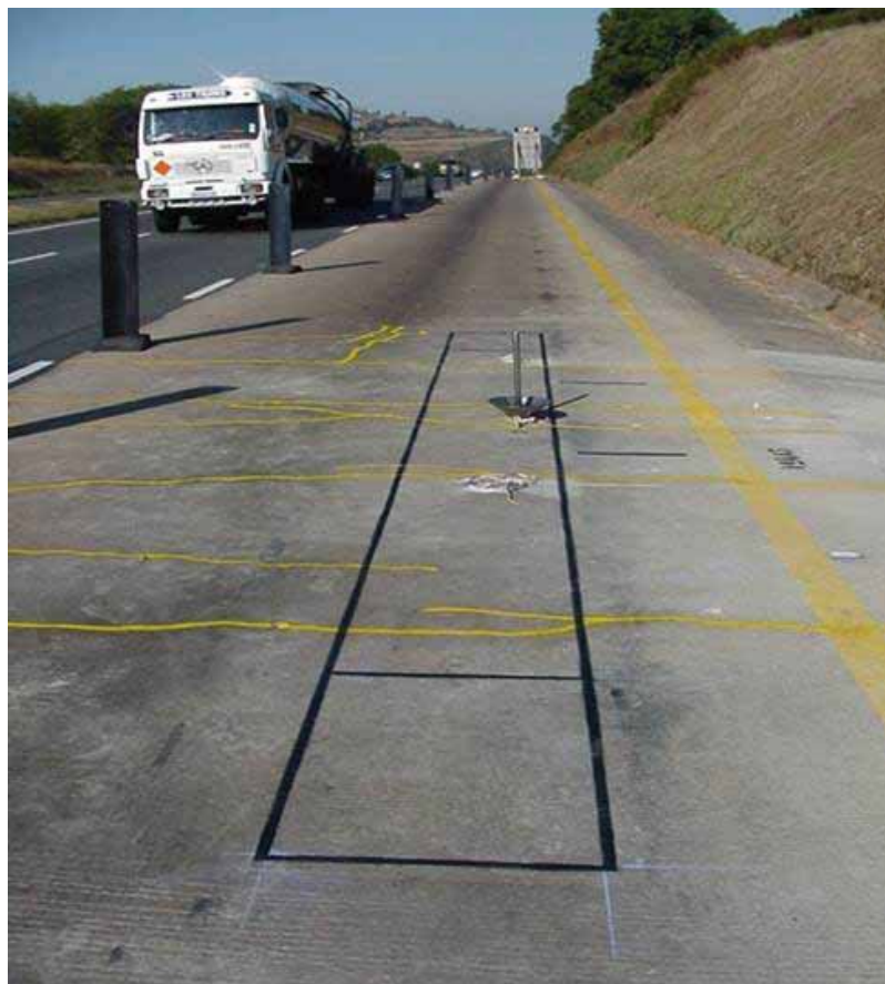
Picture 2.3: Selected area for HVS testing on the N3 concrete inlays.
