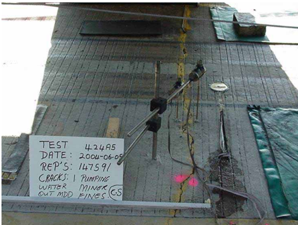
Picture 5.2: Water seeping out of the MDD holes
