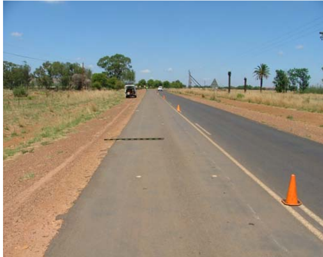
Figure 3.2: General view of H1-04-G-2388
